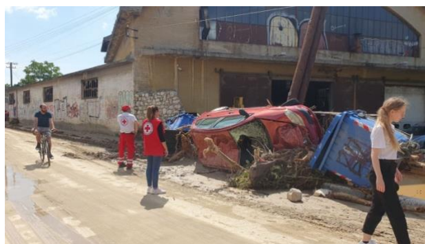
Figure 10: Flood damage in Volos, Greece, following Storm Daniel in September 2023. Credit: Greek Red Cross
